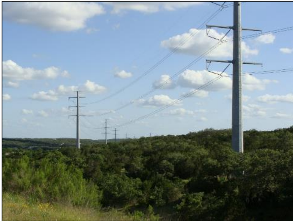
Figure 3. Typical steel monopole transmission line.
